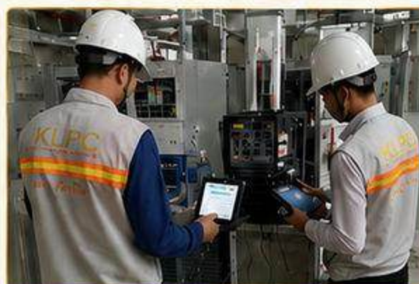
TESTING &amp; COMMISSIONING
